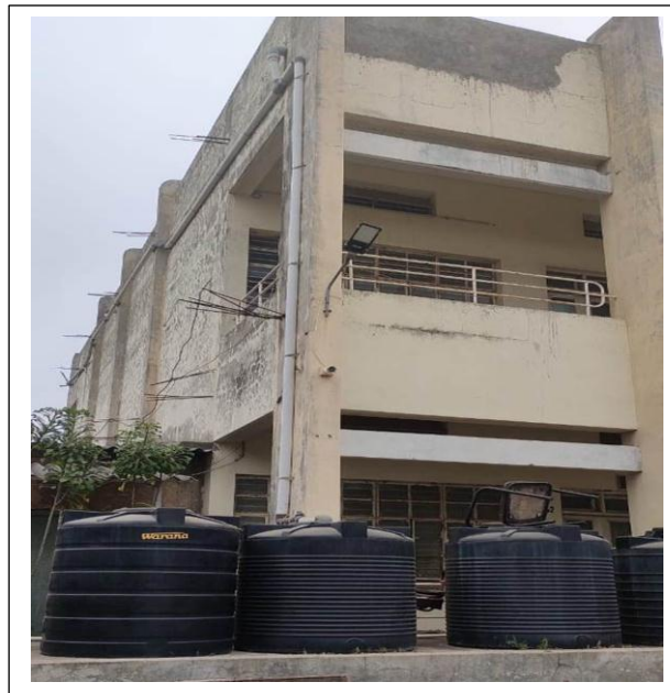
Rain Water Harvesting System
