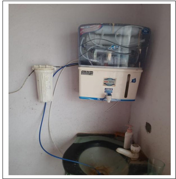
Reuse of R.O. rejected water
